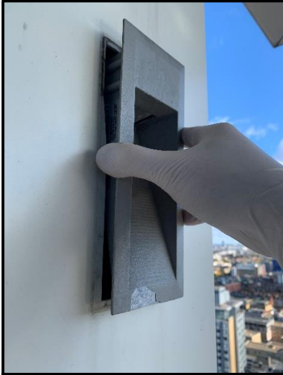
1. Remove the entire light from the cladding
