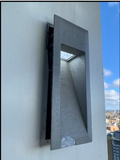
13. Turn power back on and test before fully refitting into the cladding
