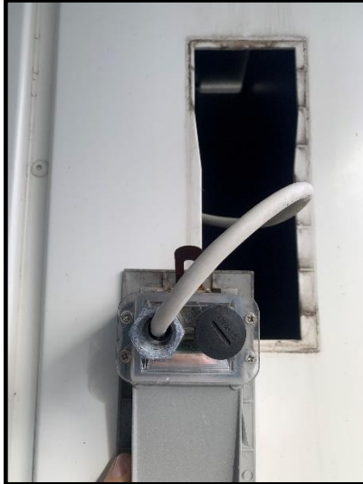
2. Remove the 4 screws and put light surround to one side
